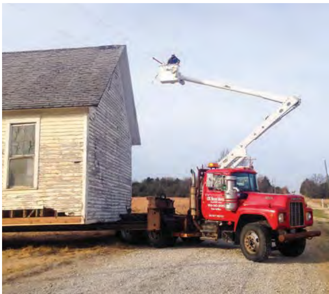
Radiant lineman, Jake Gillum raises the electric line that allows the building to move safely beneath it.
